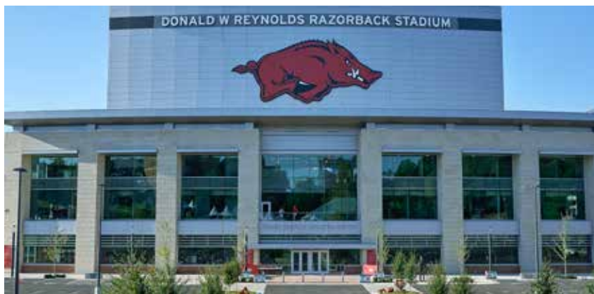
Broyles Athletic Center, in the north end, houses the athletic director and department offices.
