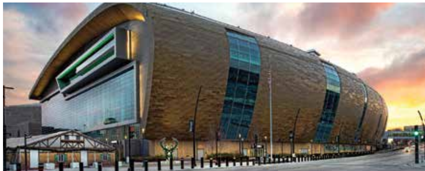
Mortenson turned over the keys to Fiserv Forum, the Milwaukee Bucks new home court, two months ahead of schedule, giving the team time to prepare for its grand opening.
