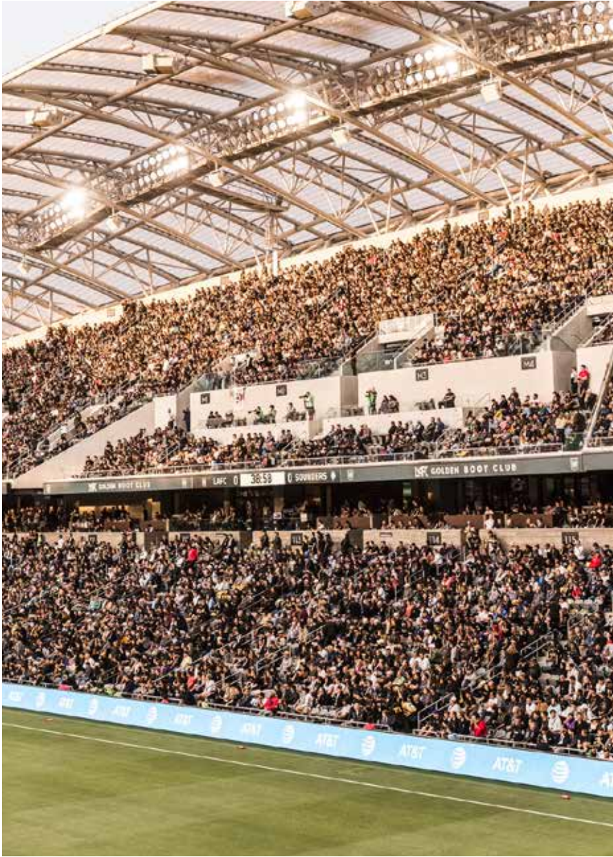
The stadium's ETFE roof reduces glare and heat on the packed stands, while leaving the field open to the California sky.
